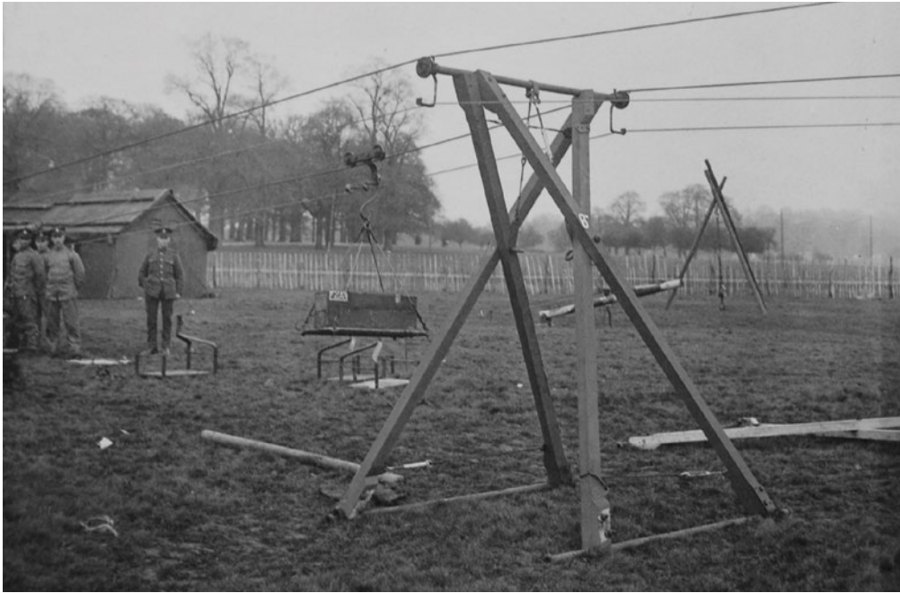
The aerial ropeway pylon © Crown Copyright
